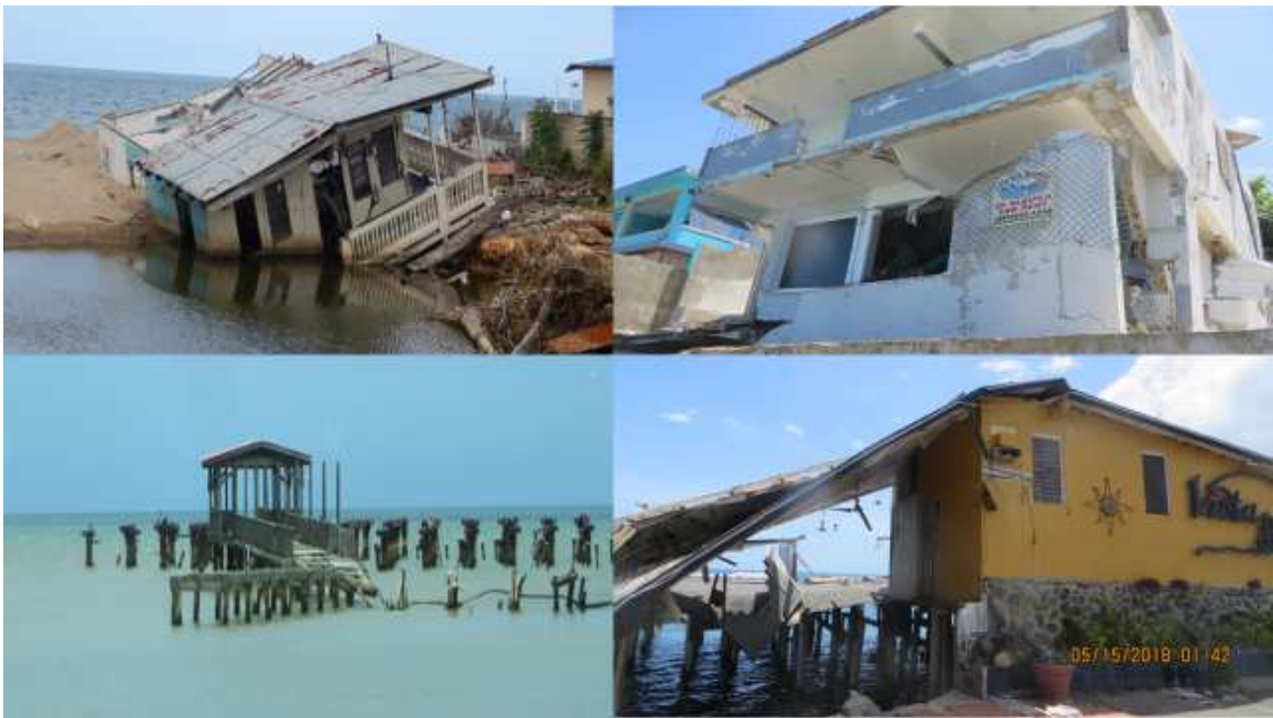
Figure 3.1: Images of structural damages captured during the field study (NSF Rapid, 2018).
