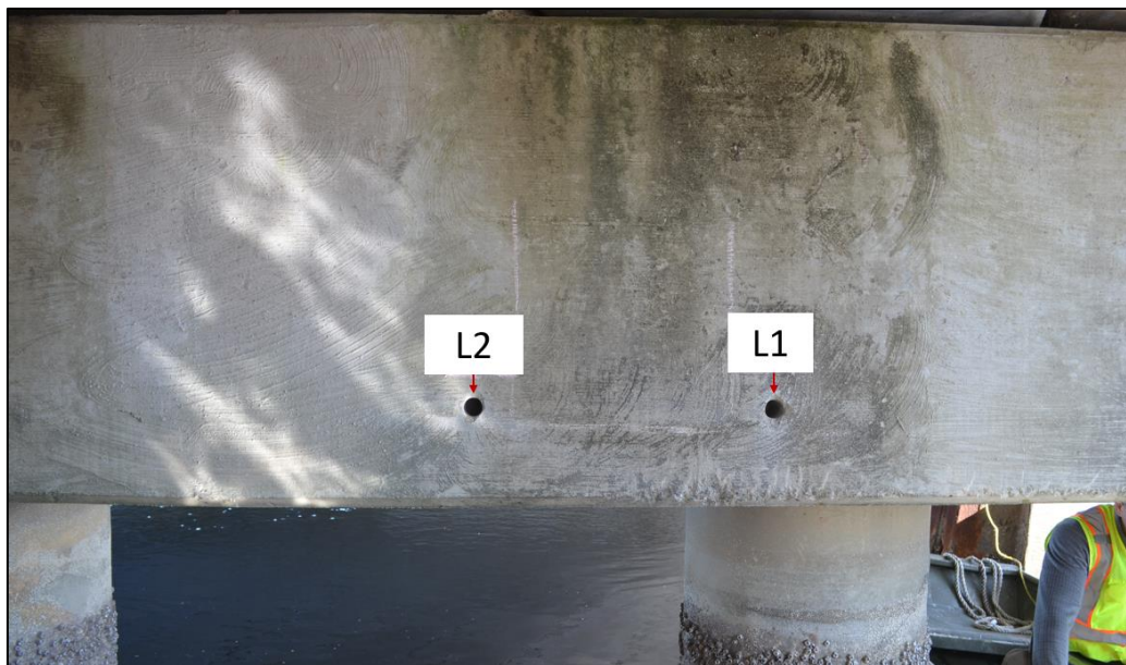
Figure 4.5: RCT test locations L1 and L2 on bridge 260007
