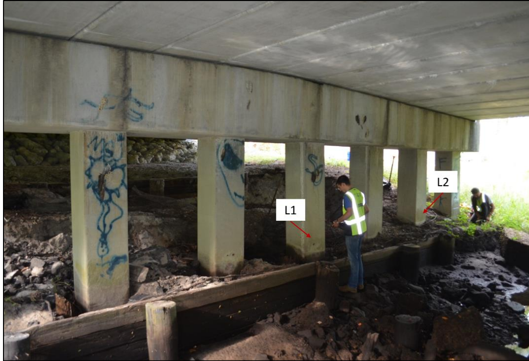
Figure 4.1: RCT test locations L1 and L2 on bridge 150020
