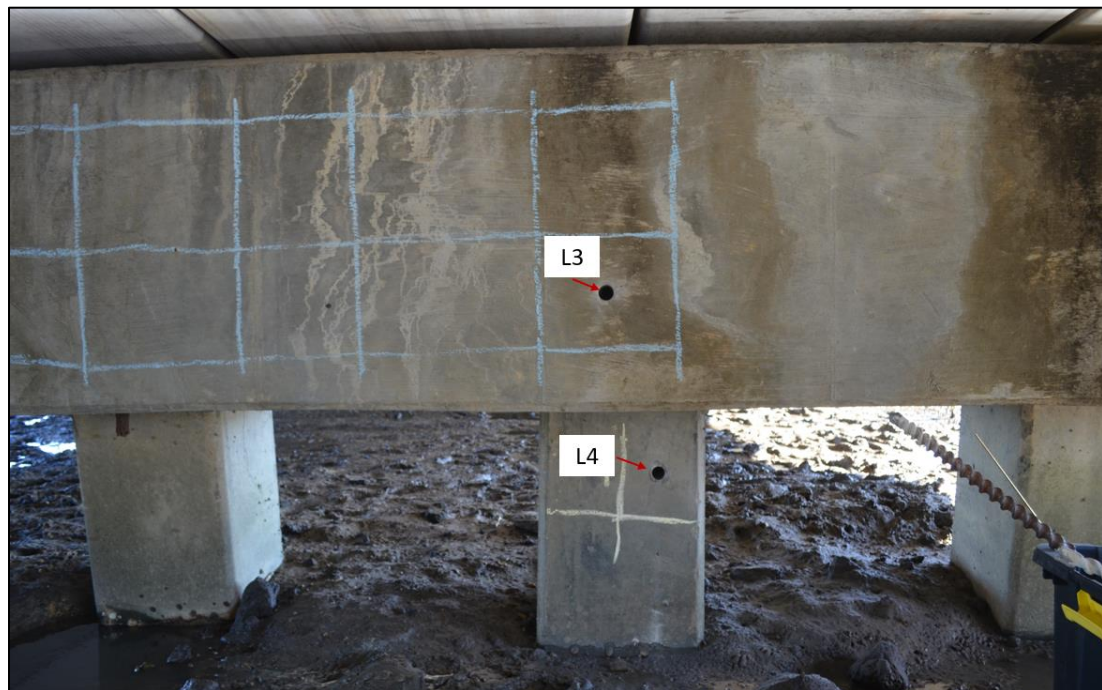
Figure 4.8: RCT test locations L3 and L4 on bridge 640010
