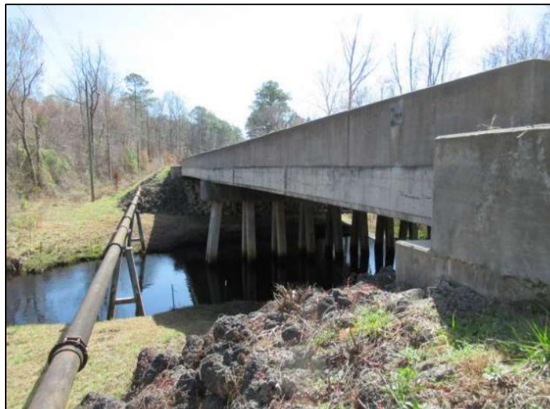
Figure 3.7: Bridge 660019 from north side
