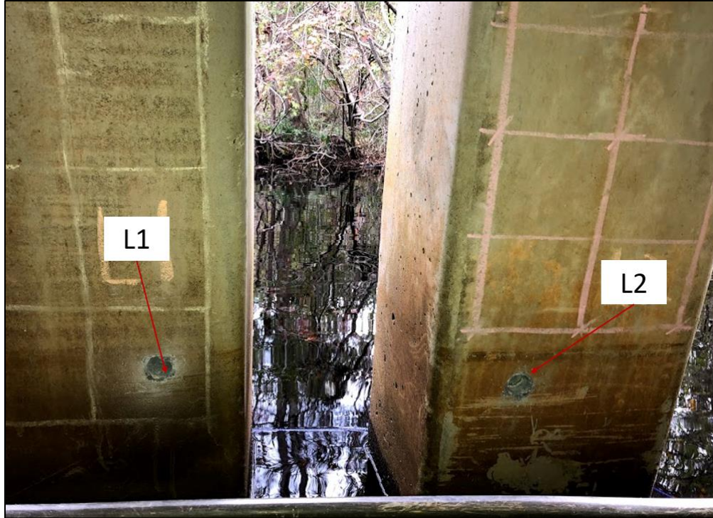
Figure 4.3: RCT test locations L1 and L2 on bridge 660019
