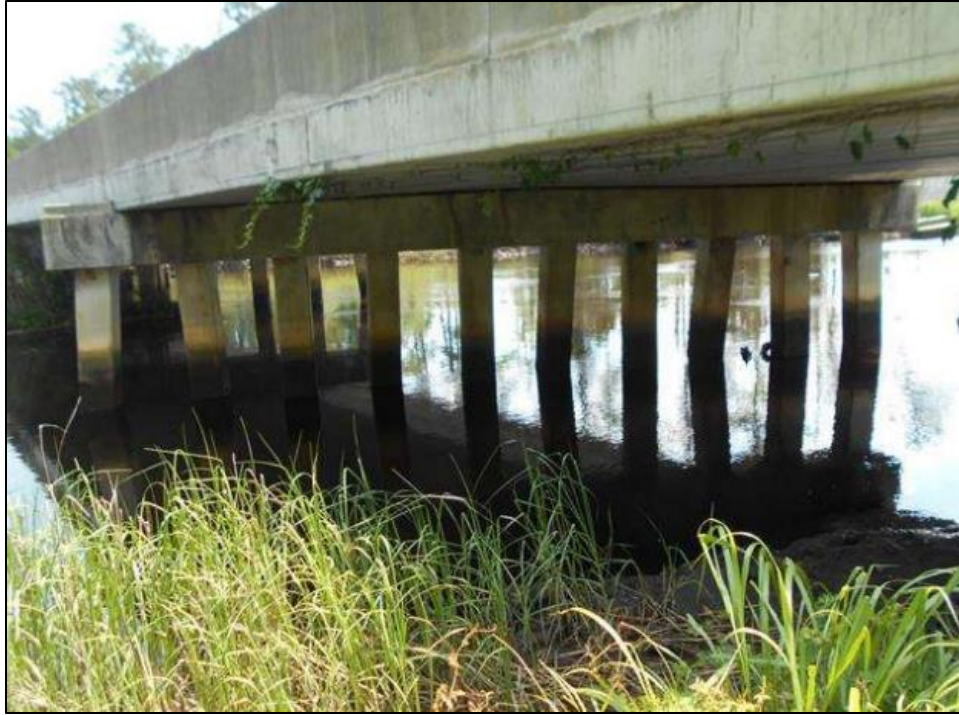
Figure 3.12: Bridge 090061 from east side
