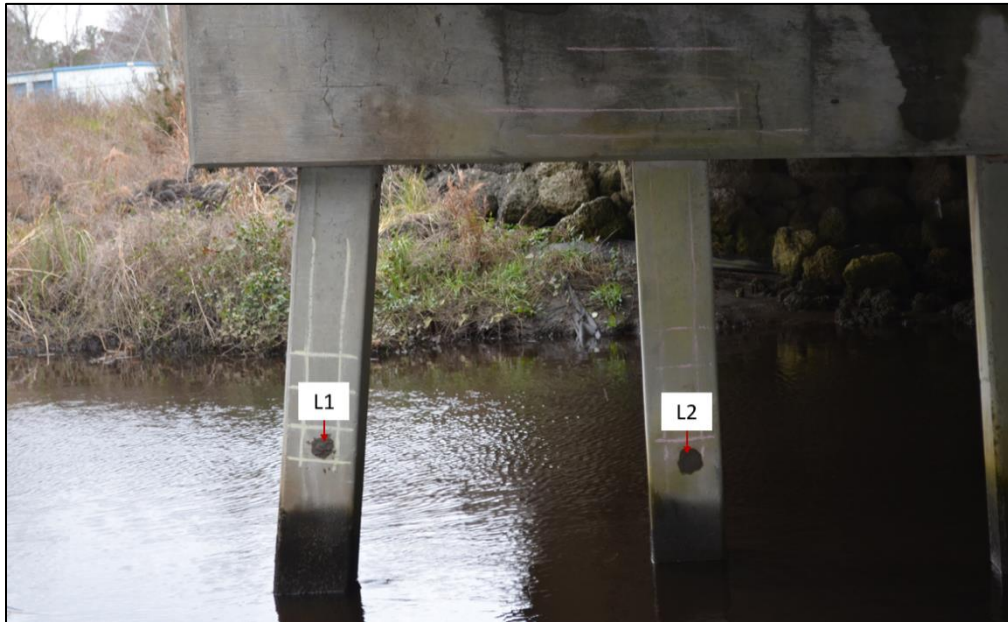
Figure 4.10: RCT test locations L1 and L2 on bridge 660021
