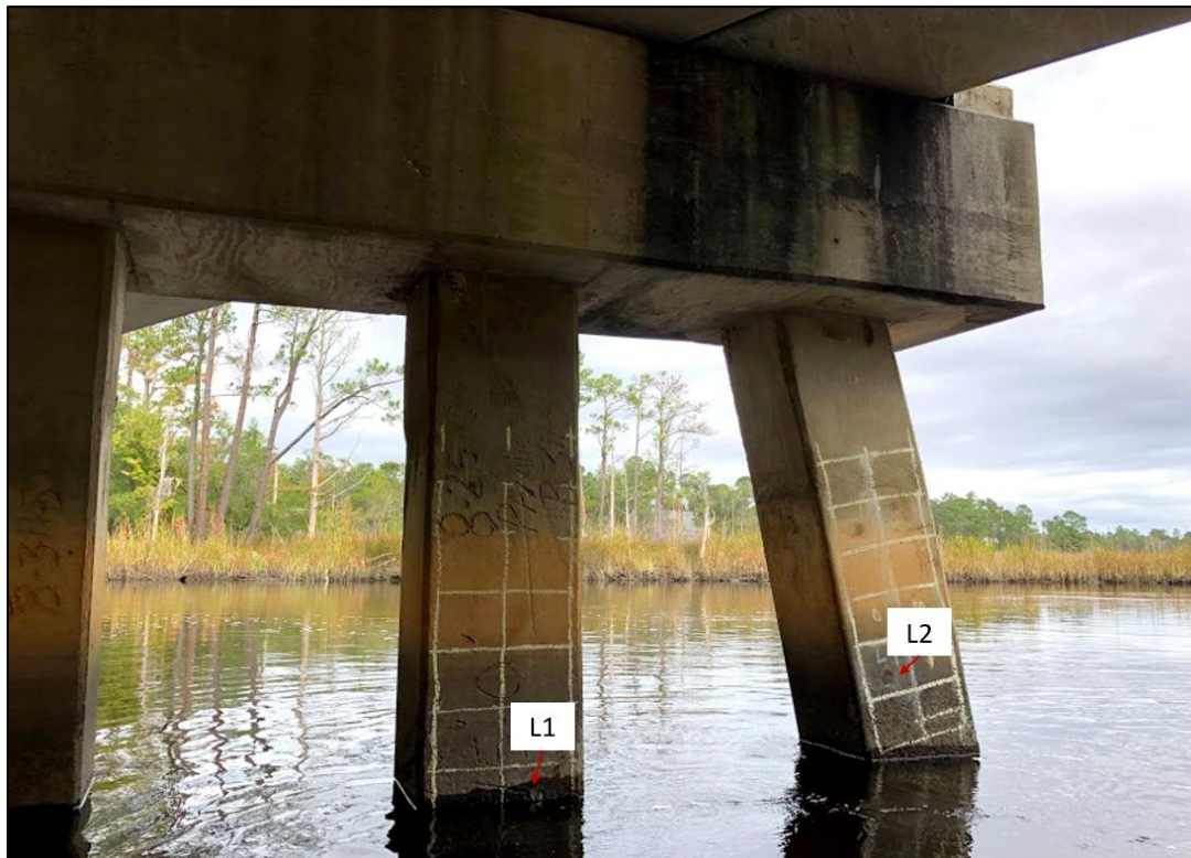
Figure 4.14: RCT test locations L1 and L2 on bridge 090061
