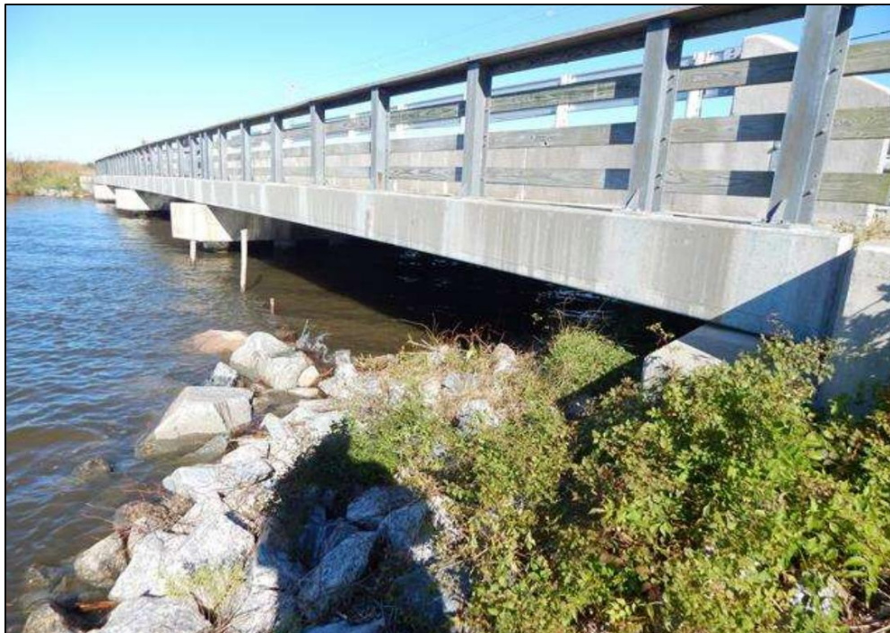
Figure 3.8: Bridge 260007 from west side
