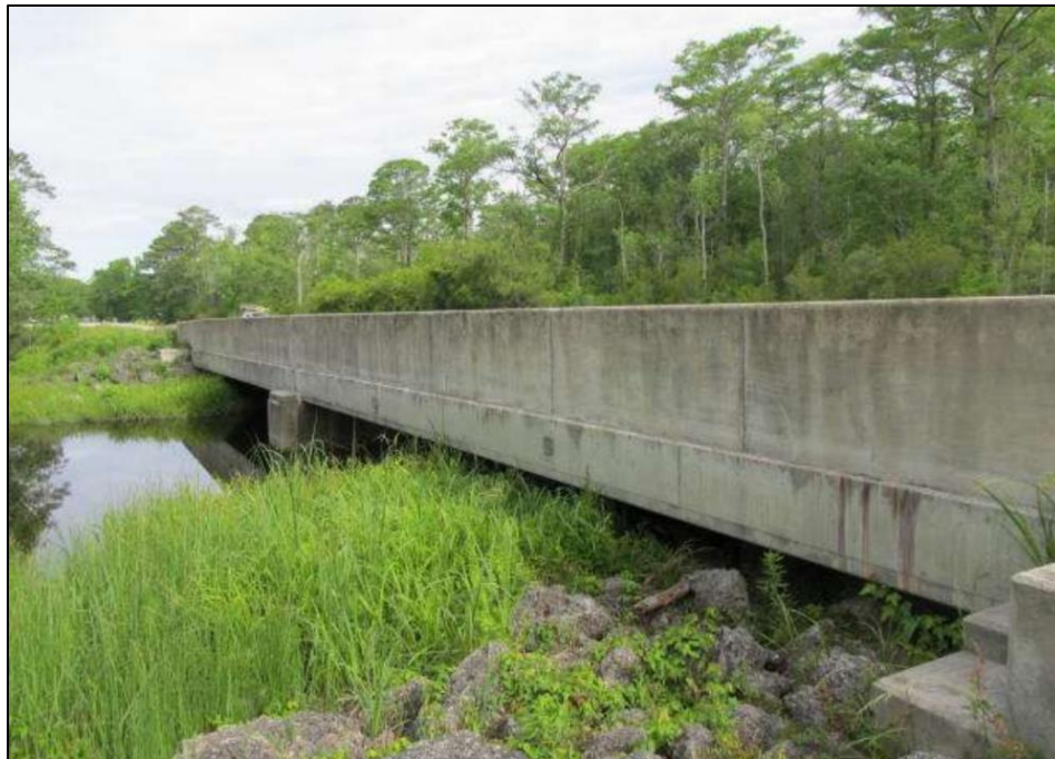
Figure 3.13: Bridge 150026 from south side
