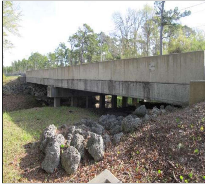
Figure 3.6: Bridge 150020 from north side
