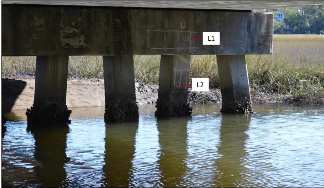
Figure 4.7: RCT test locations L1 and L2 on bridge 640010
