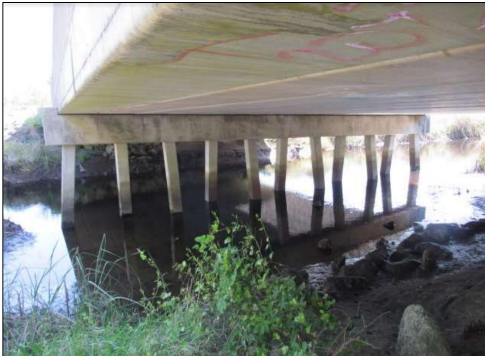
Figure 3.10: Bridge 660021 Bent 1 from north side
