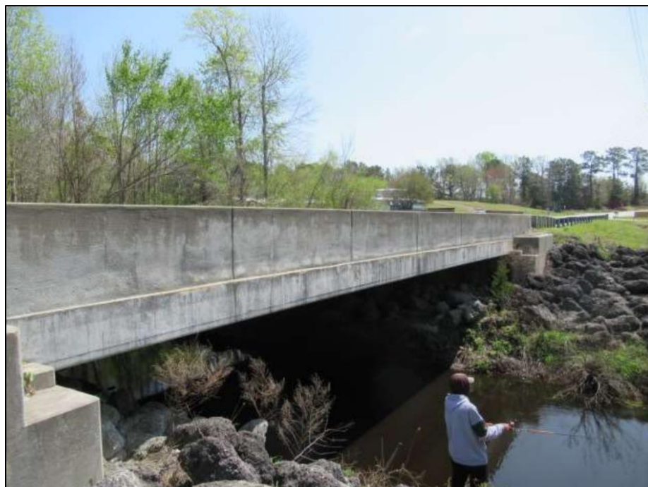
Figure 3.11: Bridge 660091 from west side
