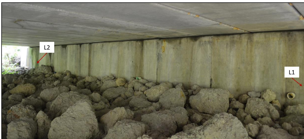
Figure 4.12: RCT test locations L1 and L2 on bridge 660091
