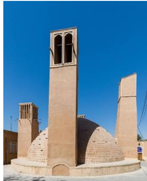
FIGURE 1 - A typical wind catcher [5]
