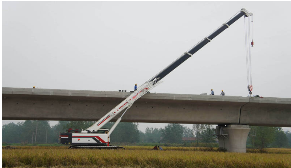
FIGURE 4: Telescopic boom crawler crane
