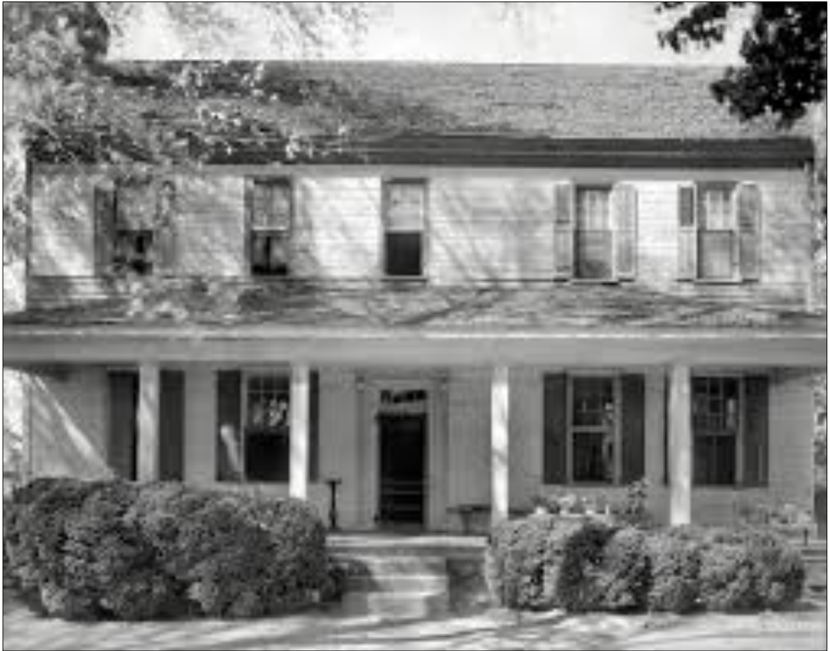
Figure 1. Photograph of Holly Bend, main house, F.B. Johnston, taken in 1938.
