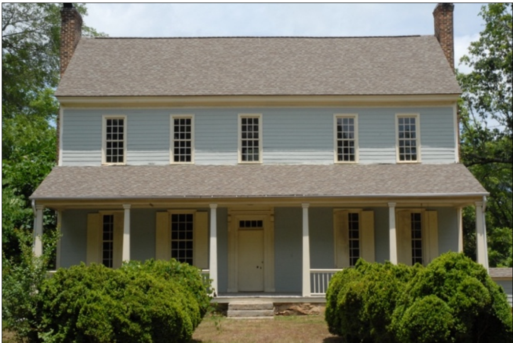
Figure 3. Photograph of Holly Bend, main house, taken by author in 2016.
