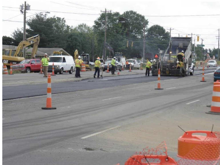
FIGURE 12: Construction workers in the median at Case Study 1
