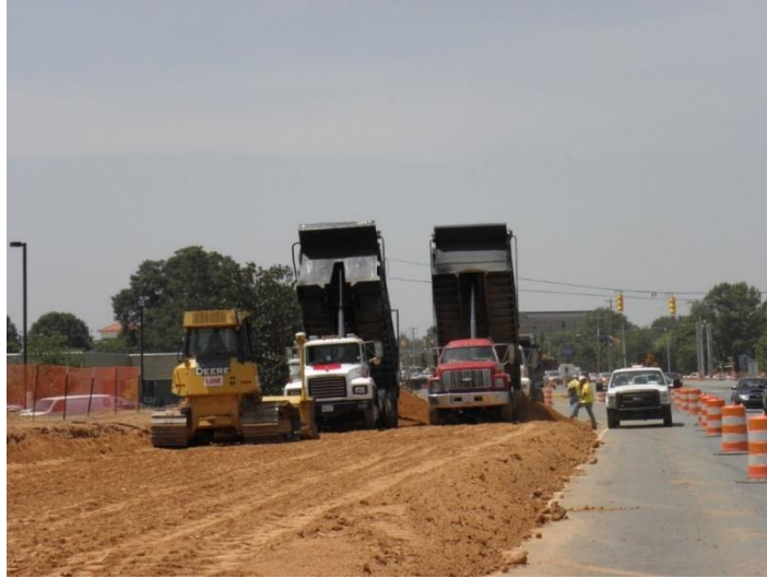
FIGURE 22: Earth work operation Case Study 3
