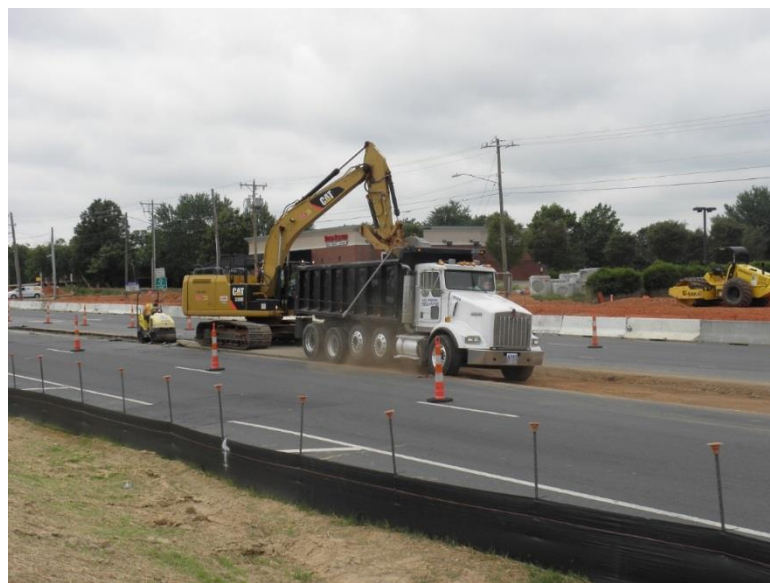
FIGURE 18: Location of work crew Case Study 2
