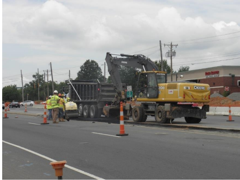
FIGURE 20: Progression of work Case Study 2
