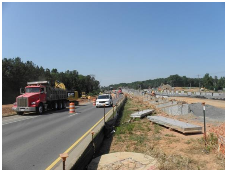
FIGURE 26: Description of work Case Study 4
