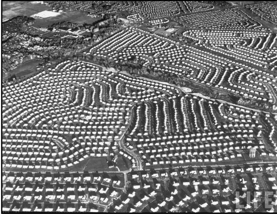
FIGURE 10: The mass expanse of new suburban sprawl can be seen in the aerial photo above. This Levittown is near Philadelphia, Pennsylvania and was constructed several years after the Levittown in New York. Source: Rollins College (2013). Photo: Margaret Bourke-White, October 1957.
