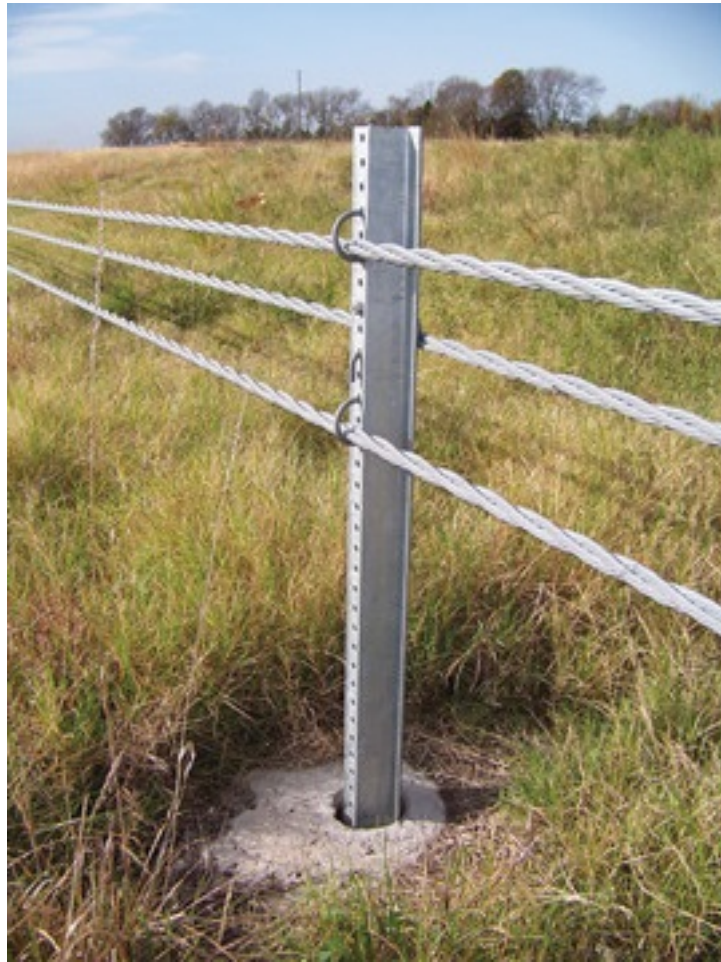
Figure 1.1: Cable median barrier.
